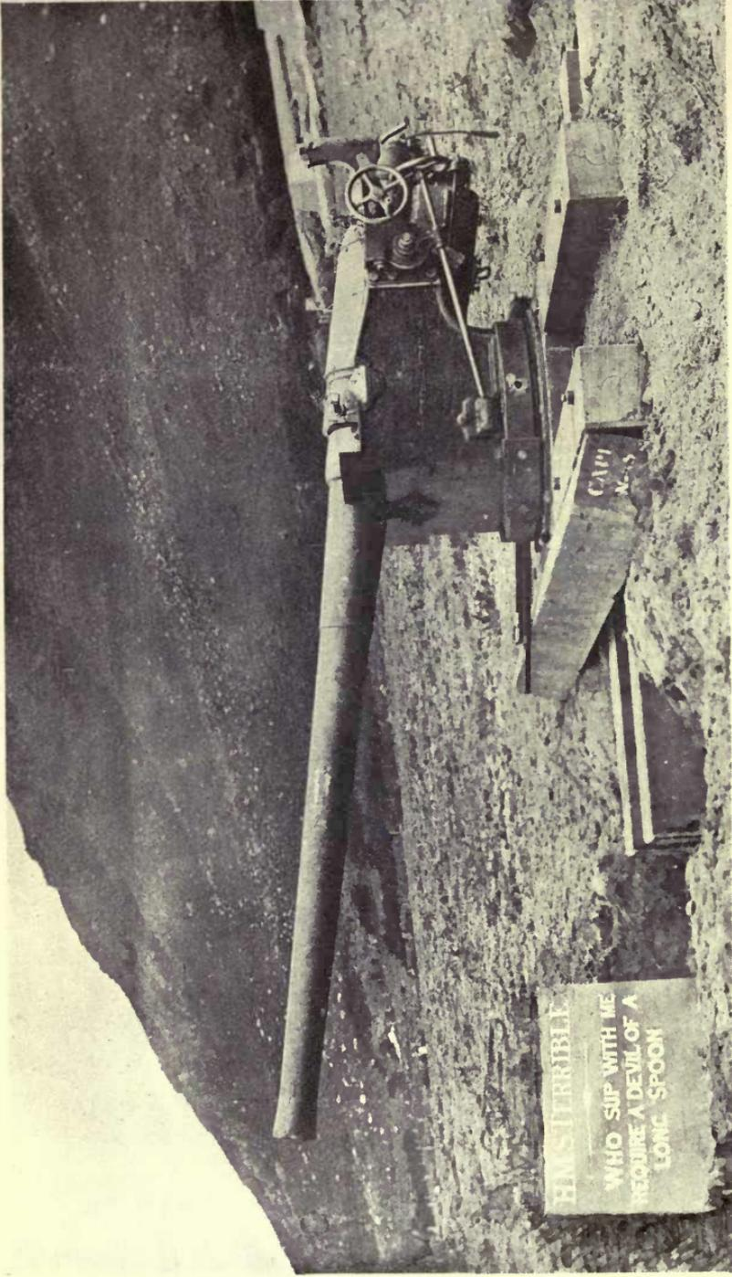
4.7-INCH GUN ON PLATFORM MOUNTING AS USED AT LADYSMITH.
